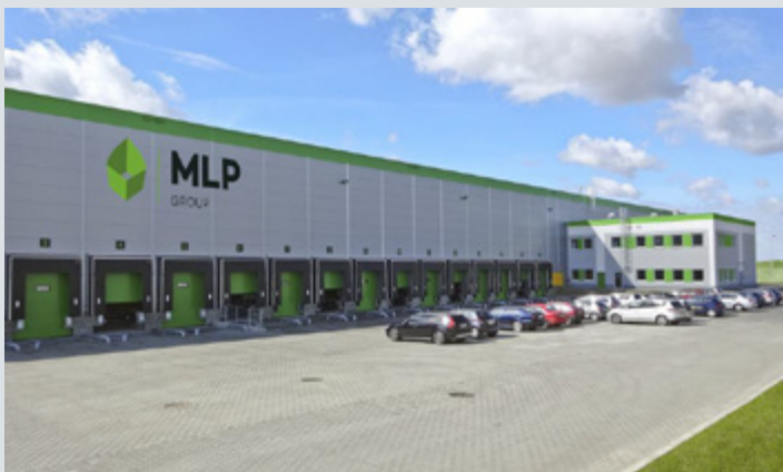
The Makro distribution center outside of Warsaw has an area of 10,100 square meters and is equipped with a dual R744 refrigeration systems for redundancy.
