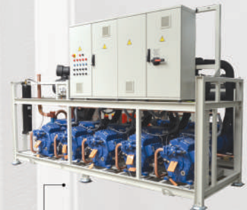
AS frame – welded frame, standard profile
