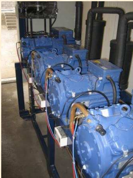
Cold store for dairy products
