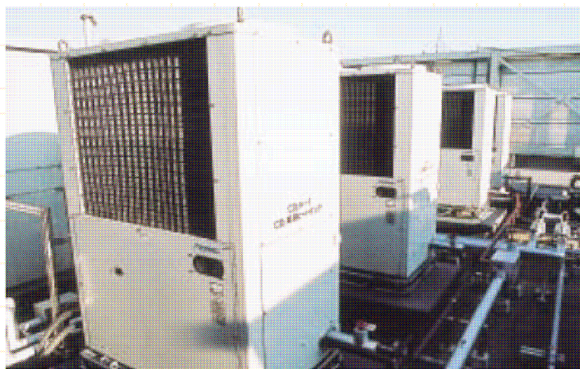
Figure 12 : Large Ecocute systems from Itomic ( www.itomic.co.jp )
