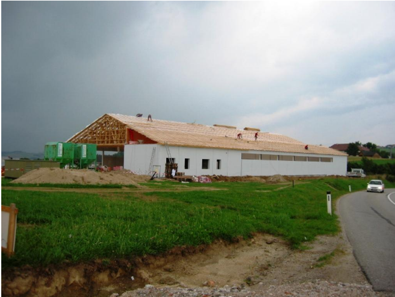
ALDI supermarket under construction
