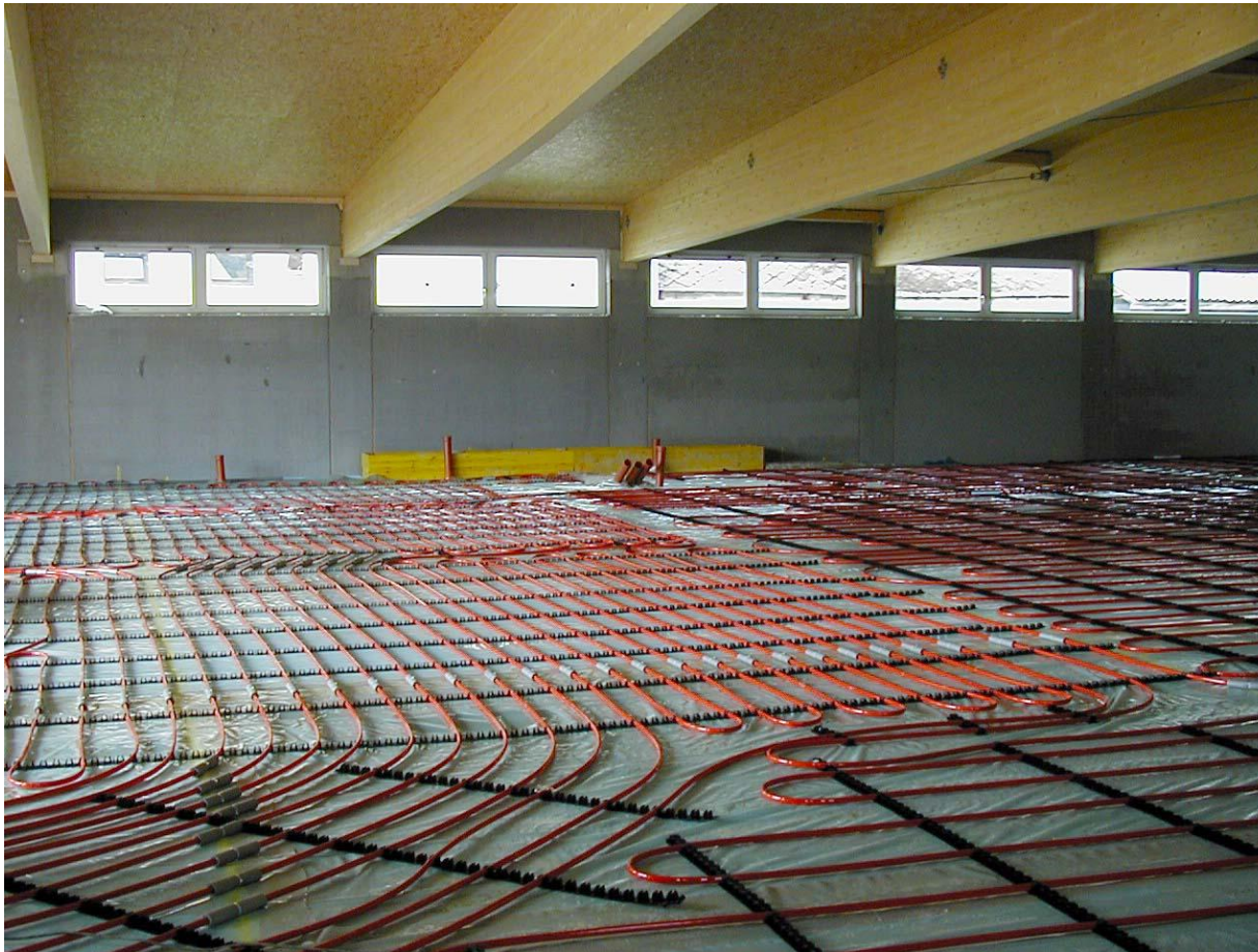
Fibre Reinforcement – Fixing with rails
