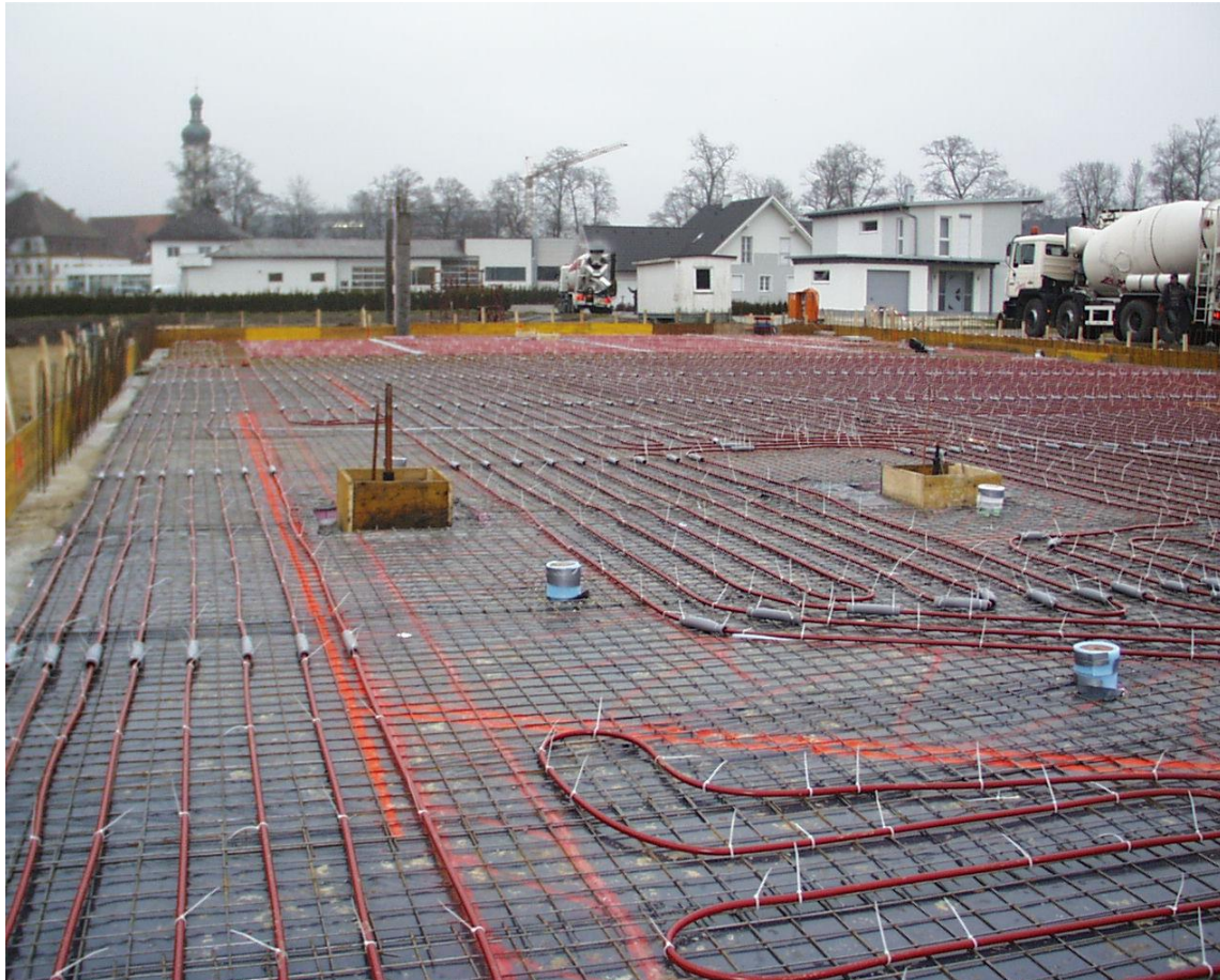
Fibre Reinforcement – Fixing with construction steel grid
