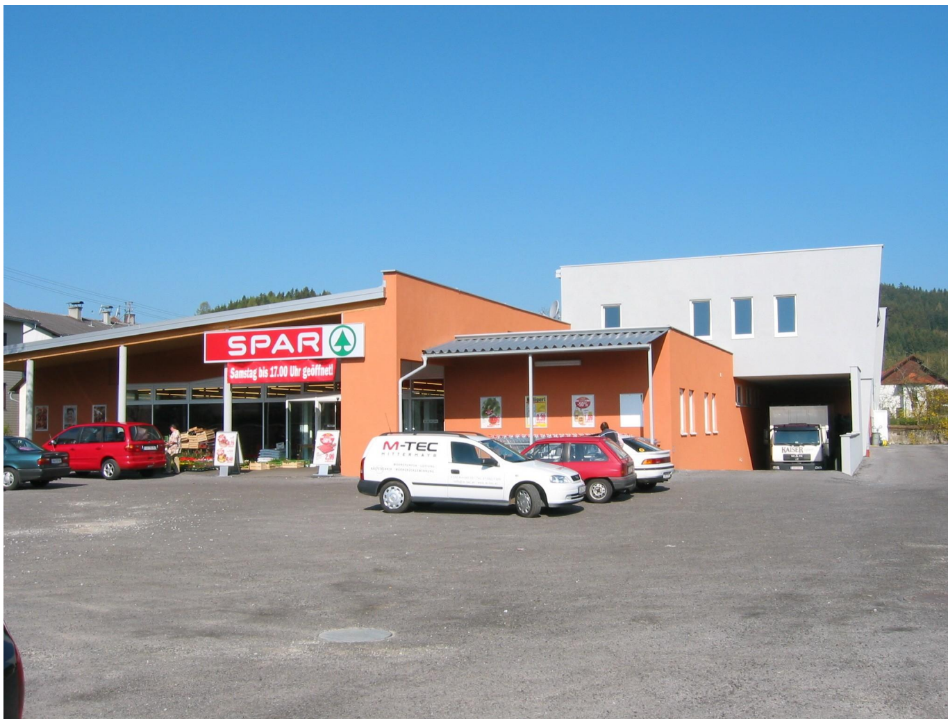
Heat recovery installation at SPAR store
