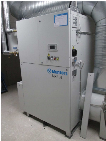
Figure 32 The dehumidifier (left) and the preheating function (right).
