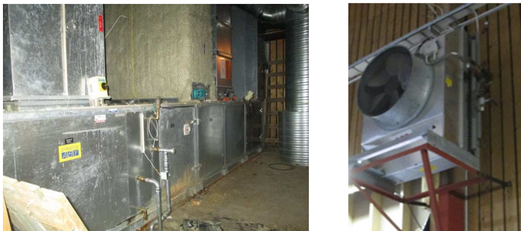
Figure 57 The ventilation unit (LB02) and fan coils units in the ice rinks space.
