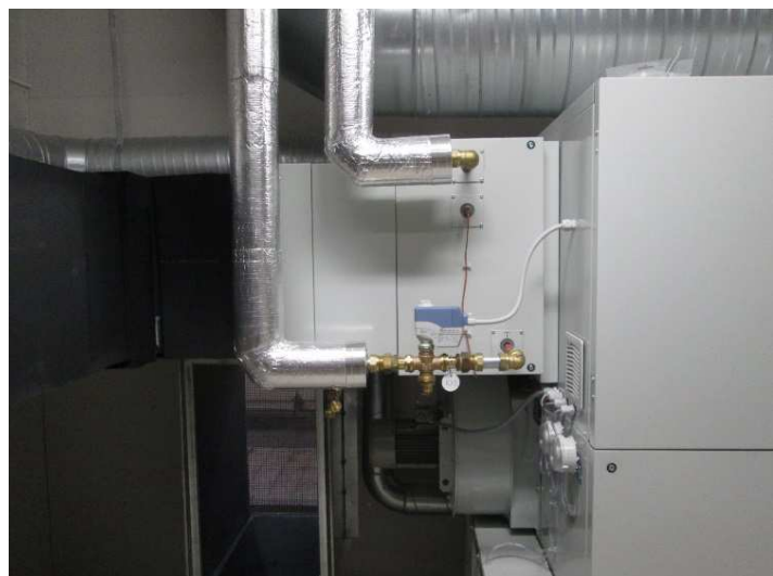
Figure 32 The dehumidifier (left) and the preheating function (right).
