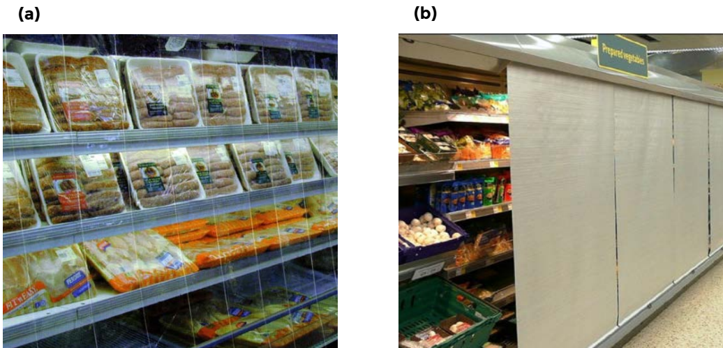
Figure 4 (a) Strip curtains (TMI International LLC, 2000) and (b) Night blinds for open front cabinet (Commercial Blinds UK Limited)
