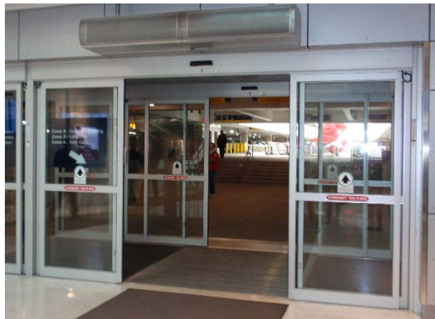
Figure 7 Vestibule entrance with two door sets and air curtain (BERNER International Corp., 2014)
