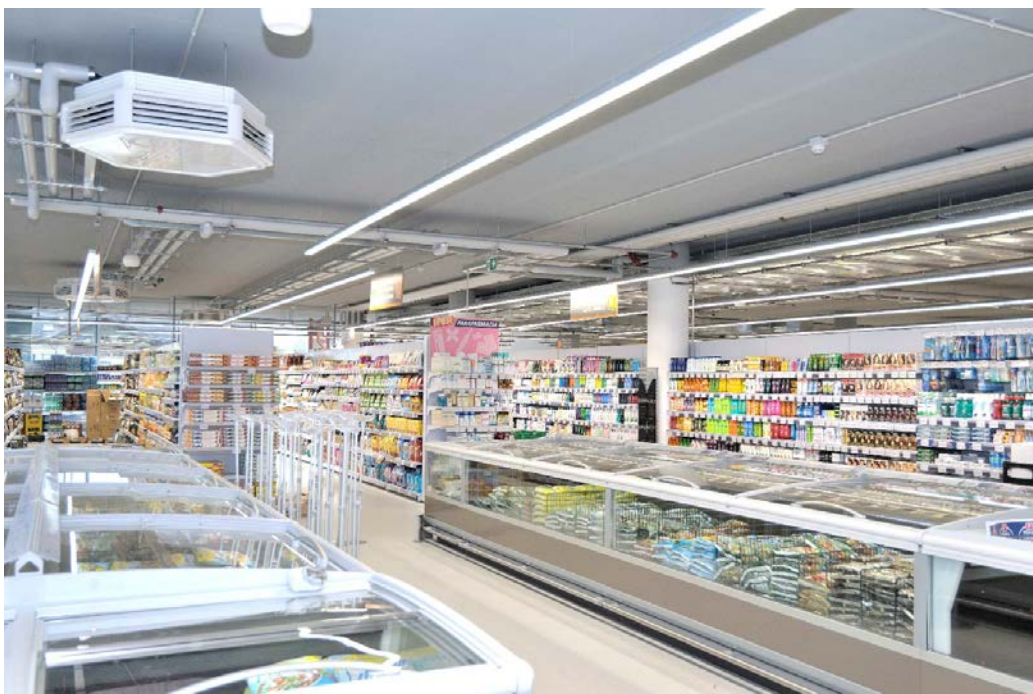
Figure 9 Local direct CO 2 heating/cooling unit by Enex (Giroto 2016).
