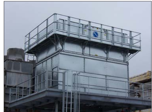
Standard Construction Installation
