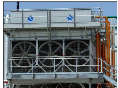
EVERTOUGH™ Construction Installation
