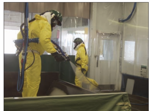
Application of TriArmor® Corrosion Protection System
