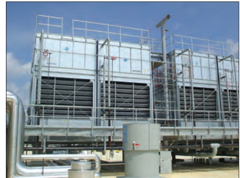
Multi-Cell CXV-T Installation Showing Simplified Piping
