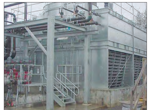
Basinless Unit Construction
