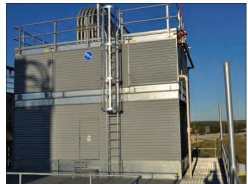
Standard Construction Installation
